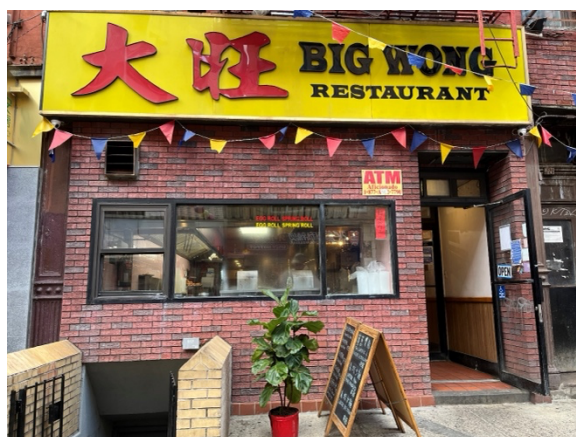
Figure 2. Lin Kwok Keung sued Big Wong Restaurant in August 2015 and settled the case in October 2017. The complaint alleged ADA violations including a step at the entrance without an ADA compliant ramp or wheelchair lift, a restroom accessible only by stairs on the lower level, and items in the restroom installed at inaccessible heights. 64 As of February 27, 2023, the step preventing wheelchair access to the restaurant remains unchanged.
